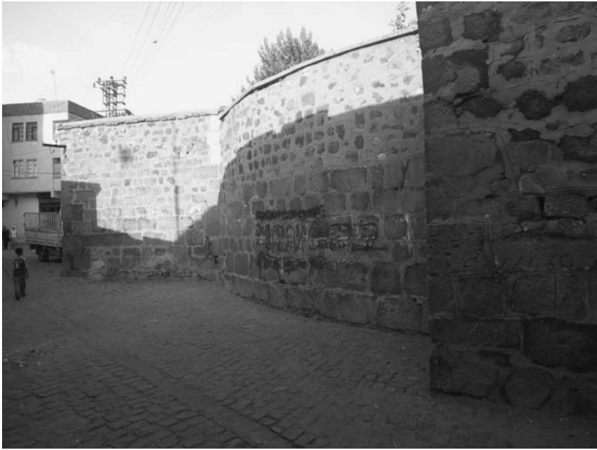
Fig. 2.4.4 Outer walls of the Church of Yoldath Alohó
